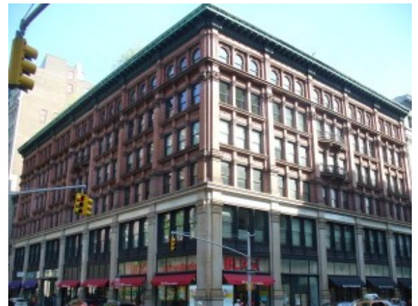
LPC approved rehabilitation, Ladies' Mile Historic District. Perkins Eastman, 2007 | Photo By: Gregory Dietrich, photographer, 6/15/14.
