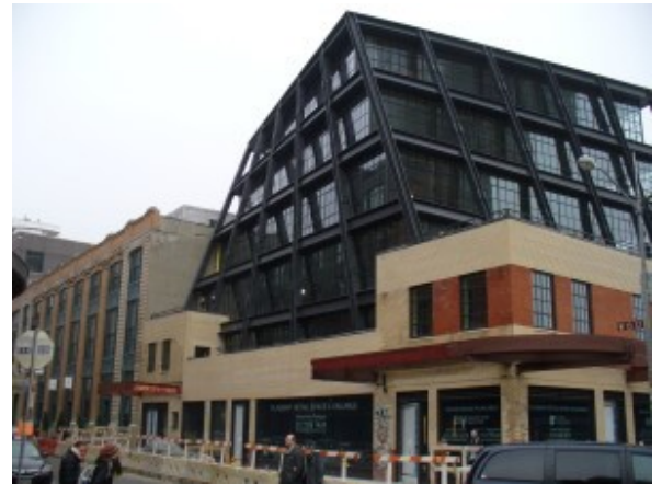
LPC approved rooftop addition, Gansevoort Market Historic District.
