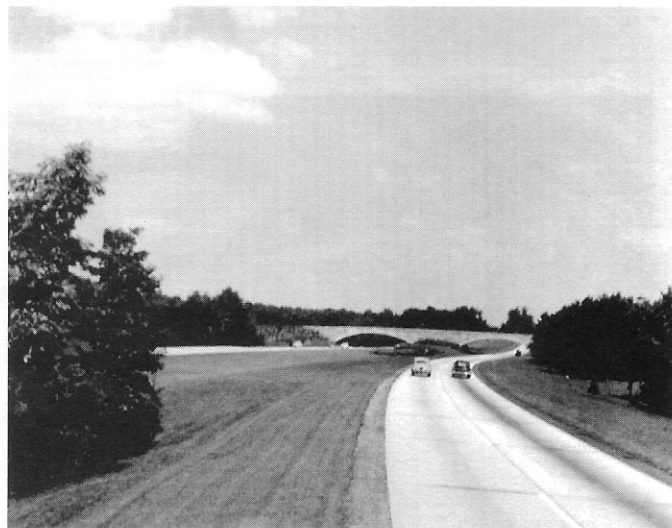
The Essex County section of the Garden State Parkway featured low-sprung, stone-faced bridges and wide, grassy medians.
