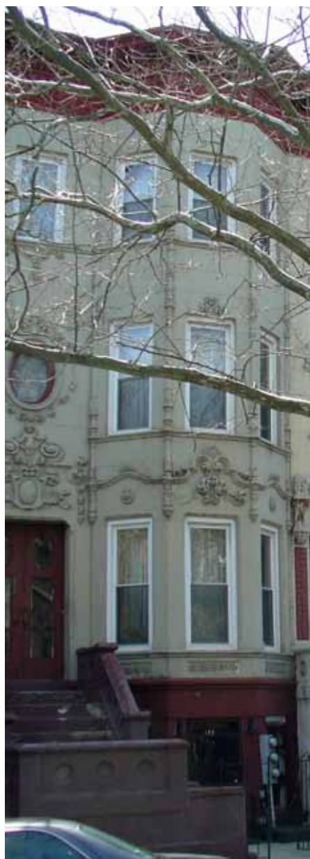
Addresses 872 to 880 on Park Place in the Crown Heights section of Brooklyn
