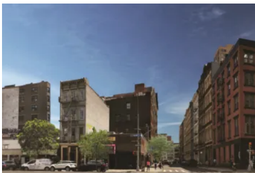
Existing building at 31 Lispenard Street./Image Credit: GF55 and Urban Standard Capital
